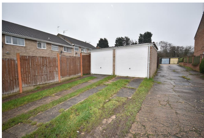
Garage and Driveway
